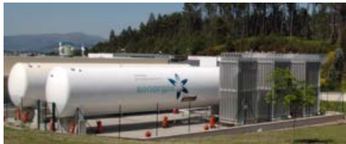
Figure 45 - Satellite Plant with Regasification Unit; courtesy sonorgás
